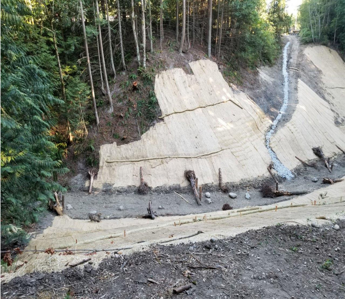
Figure 3. August 2020 Culvert now gone, and new channel opened up.
